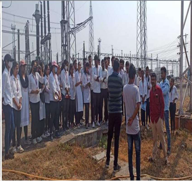
Field visit at 220kV Bale substation
